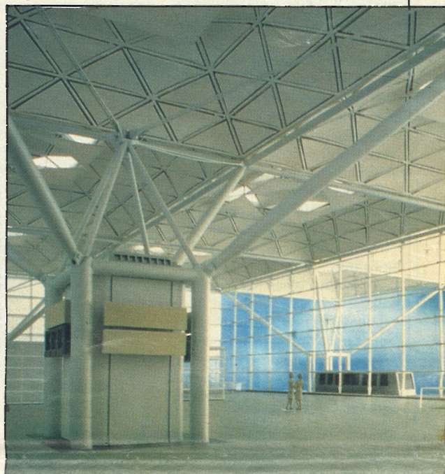
Service distribution shaft contained within a cluster of steel columns.
